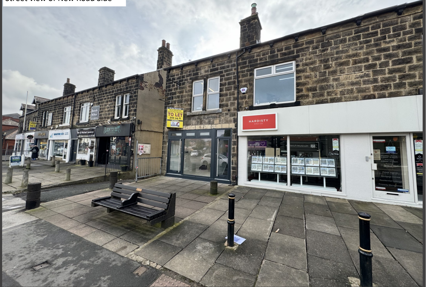
Street view of New Road Side
