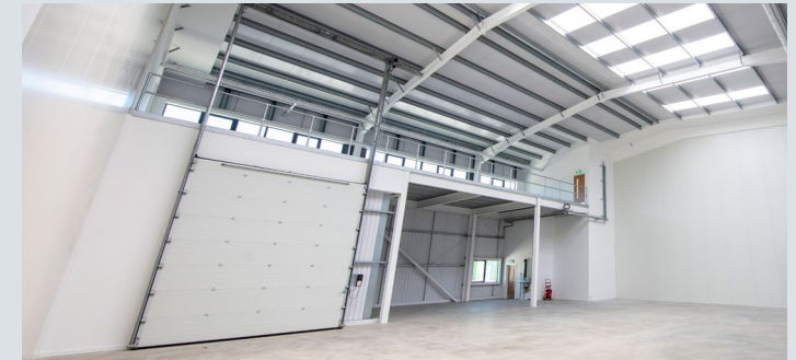
Example of fitted office
