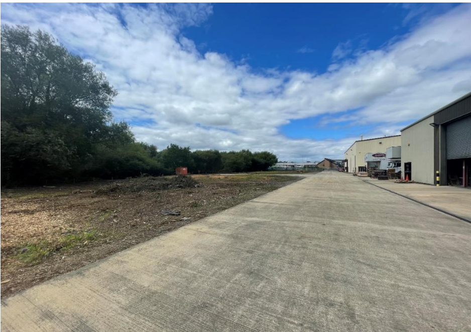
Access road looking towards front
