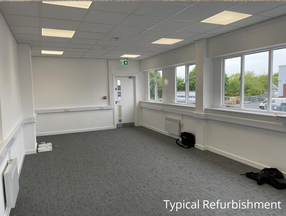
Unit 3 Avonside – Refurbished August 2021
