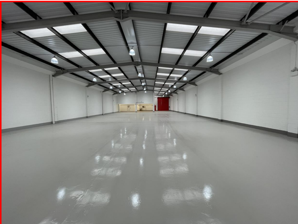
Warehouse Area Showing New Roof, LED Lighting and Painted Floor
