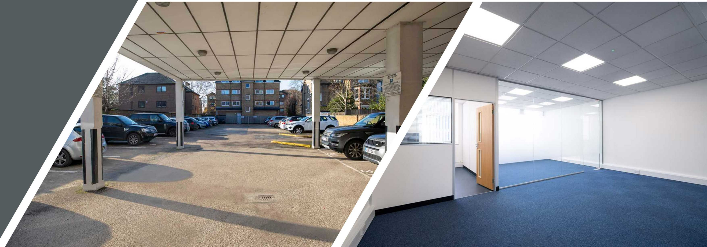
Photograph shows recently refurbished and let space.
