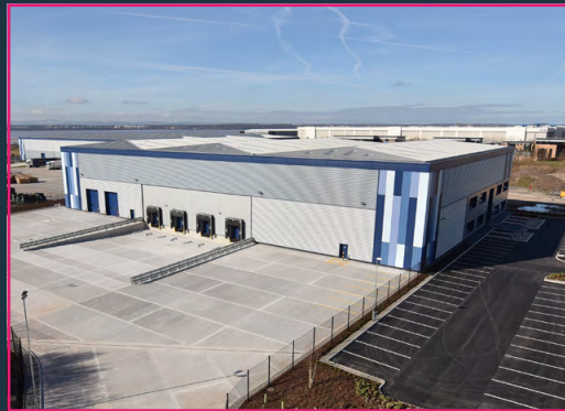
HURRICANE 52 Estuary Business Park, Liverpool
