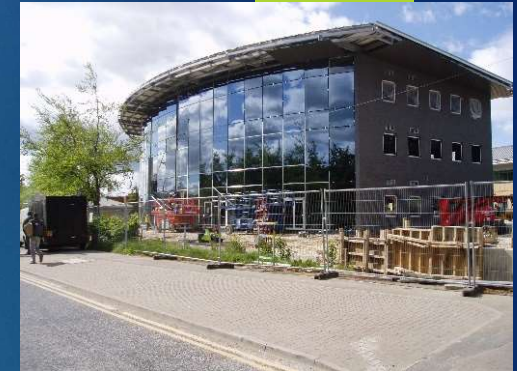
Facilities at Hornbeam Park
