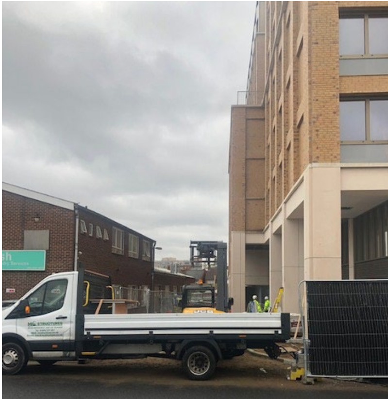
Existing Western Boundary from Palmerston Road
