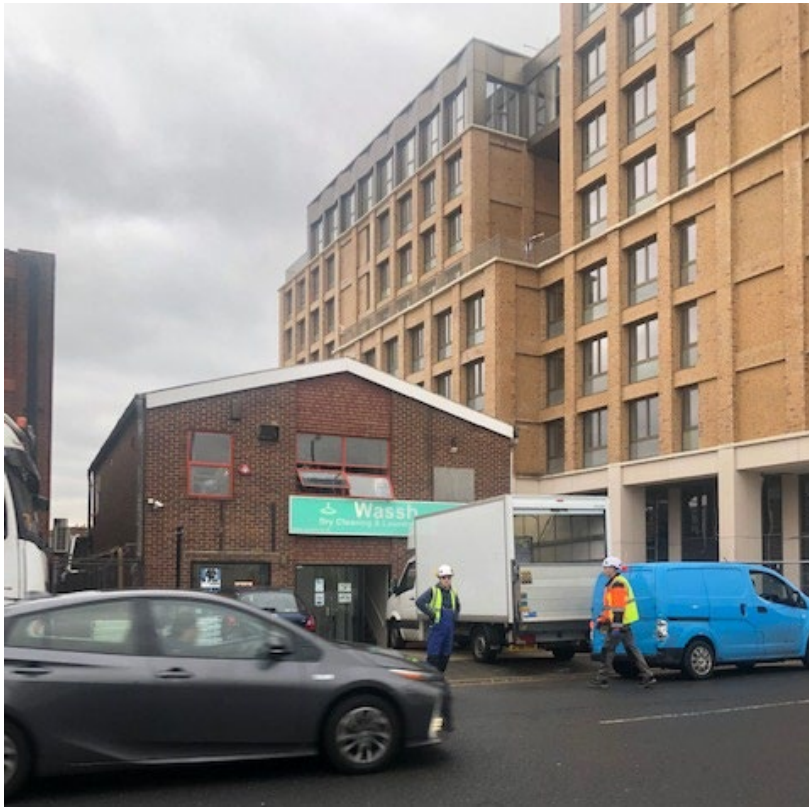
View of the existing principal elevation
