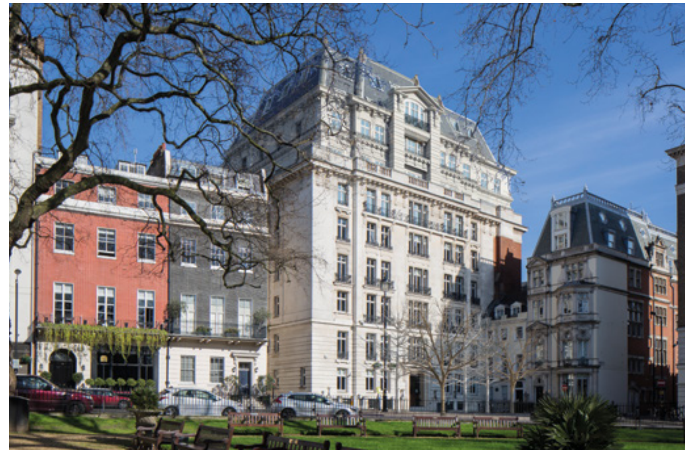
Extended storeys at 25 Berkeley Square, 56,466 sq ft, completing Q1 2020
