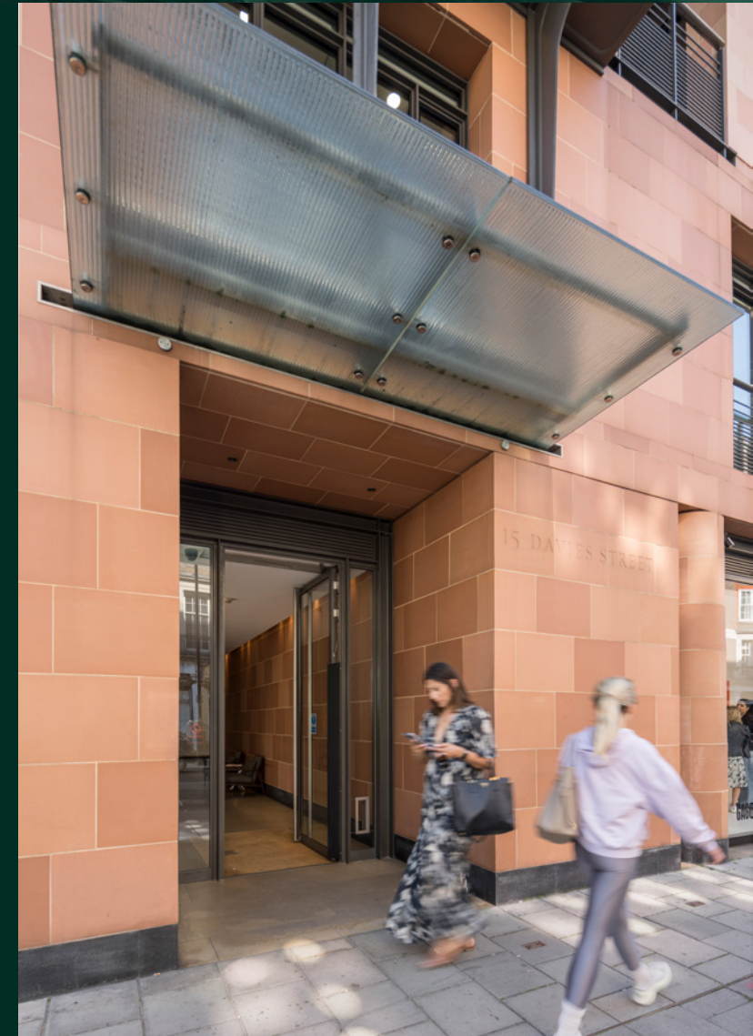
Self contained entrance
