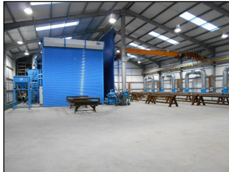
Paint Shop Interior with Crane:
