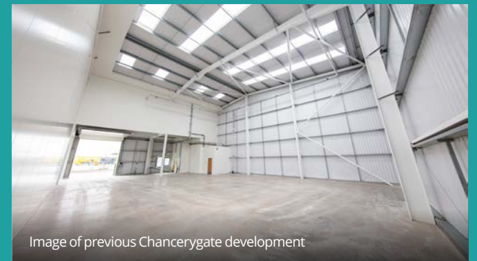
Image of previous Chancerygate development
