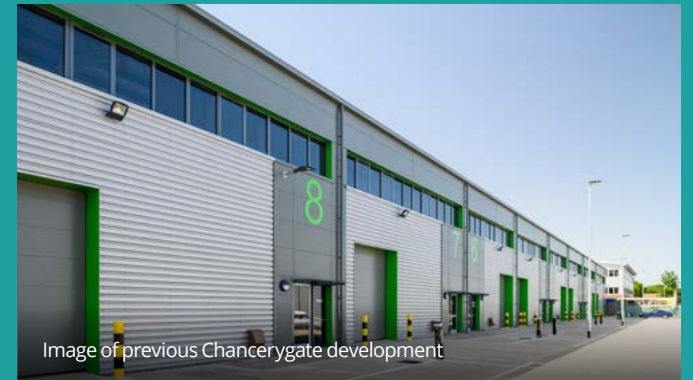
Image of previous Chancerygate development
