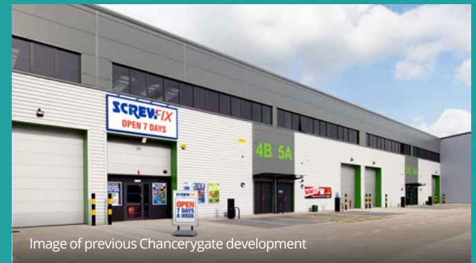
Image of previous Chancerygate development
