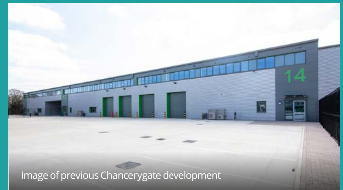
Image of previous Chancerygate development
