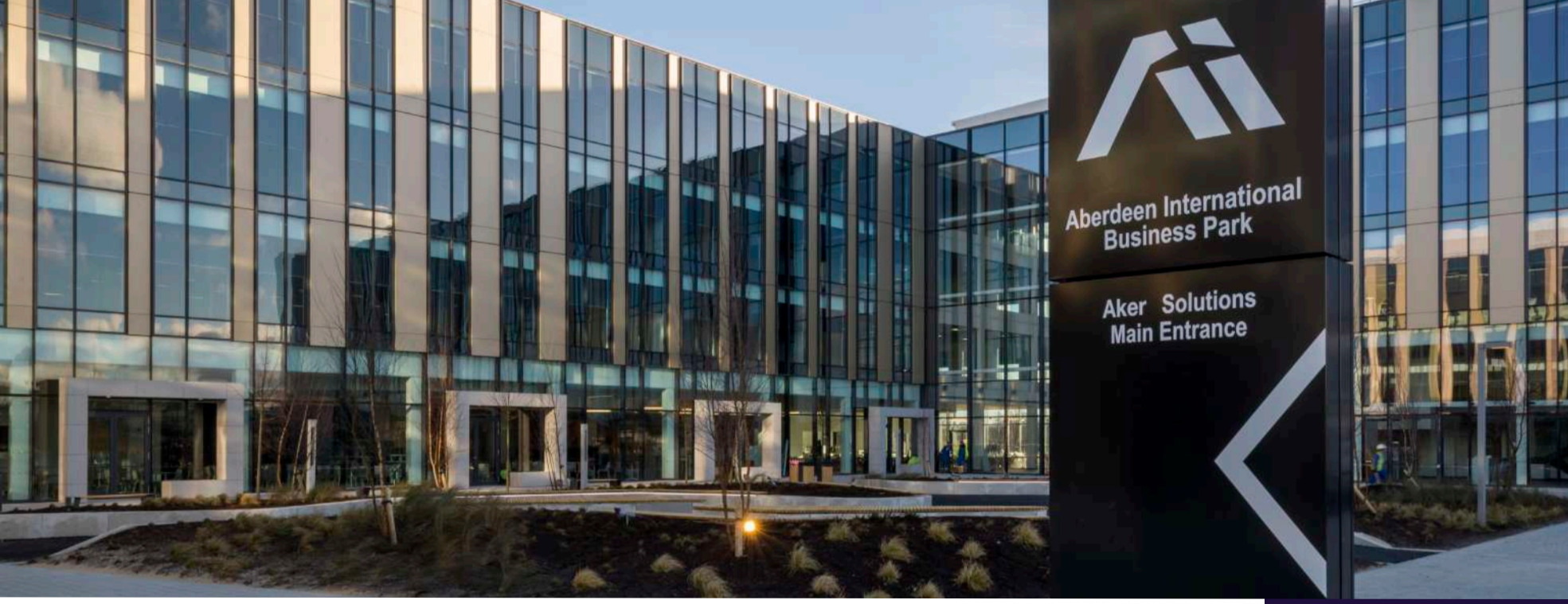
Aberdeen International Business Park (AIBP)
